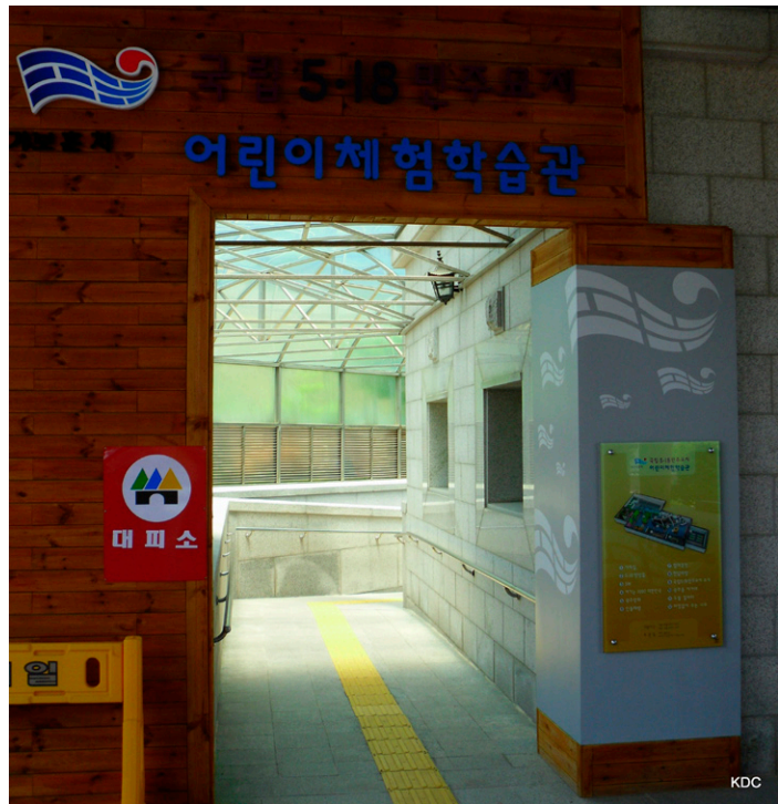
Entrance to the “children’s learning through experience hall” (어린이체험교육관) at the May 18 Cemetery. In the top left corner the logo of the MPVA which runs this hall. (May 2010)
